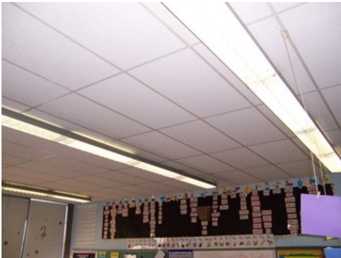
Typical Classroom Lighting
