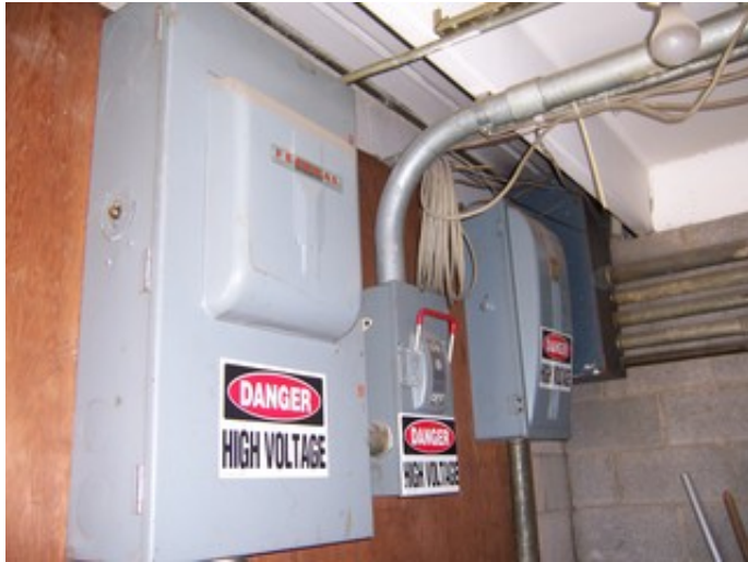
Main Utility Switch
