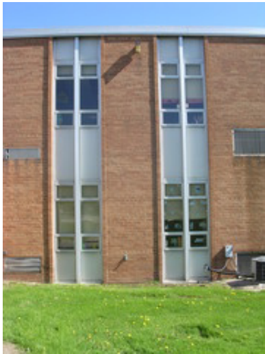
Typical aluminum windows.
