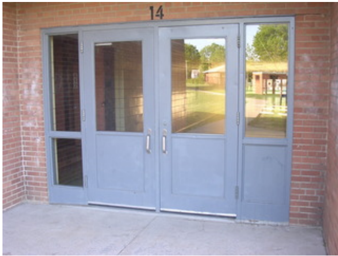
Typical hollow metal entry doors.
