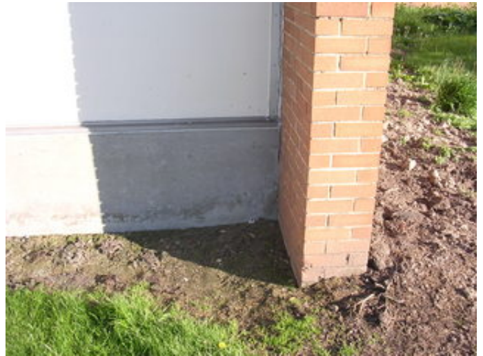
Typical foundation condition.
