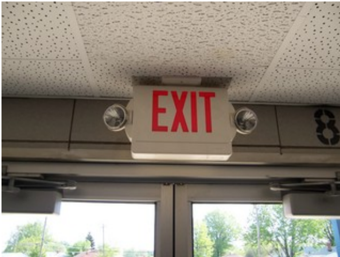
Typical Exit Sign
