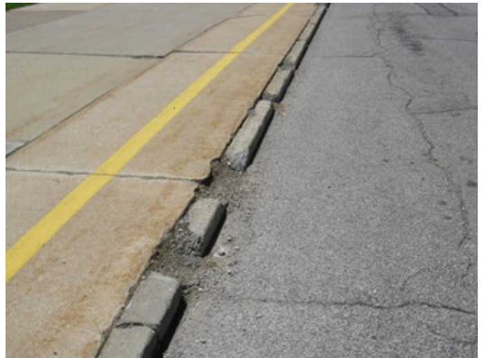
Curb in poor condition
