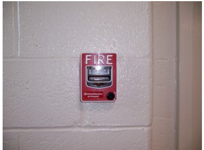
Typical Manual Pull Station
