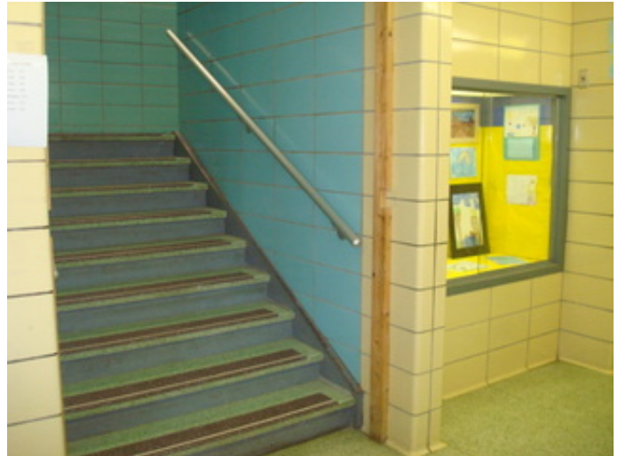
Stair and non compliant handrail
