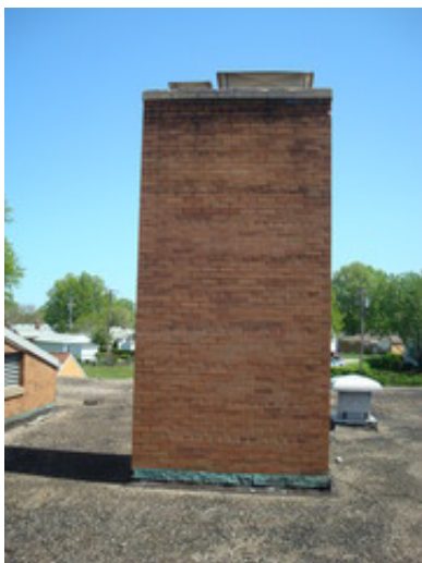
Chimney at 1956 Original Construction
