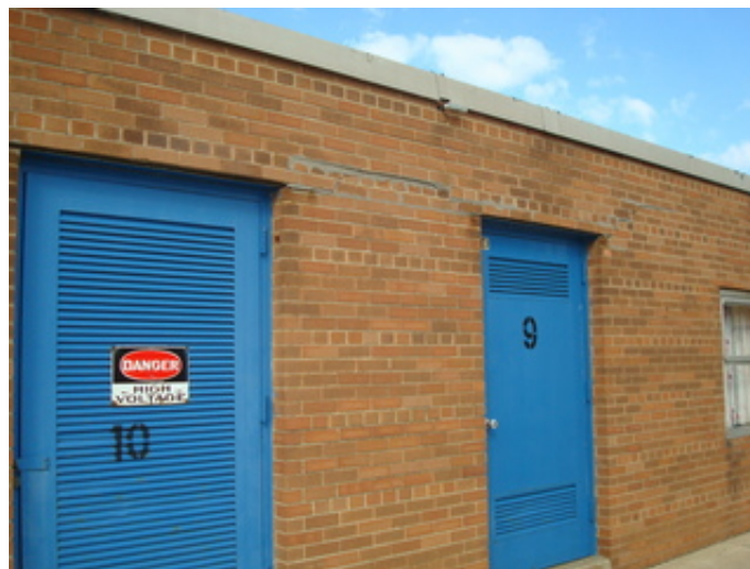
Damaged lintels and brick at 1956 Original Construction
