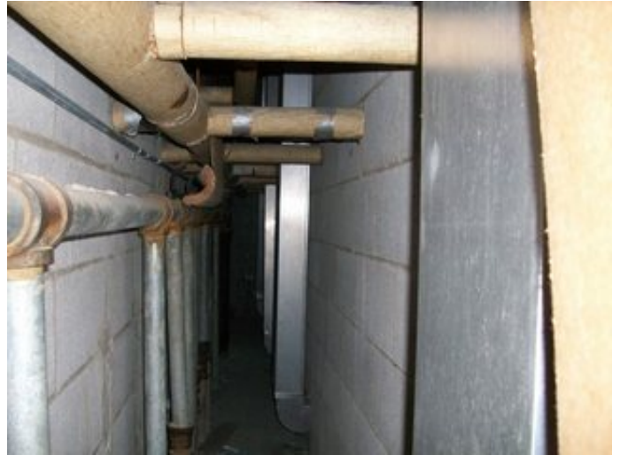
Sanitary drainage Piping
