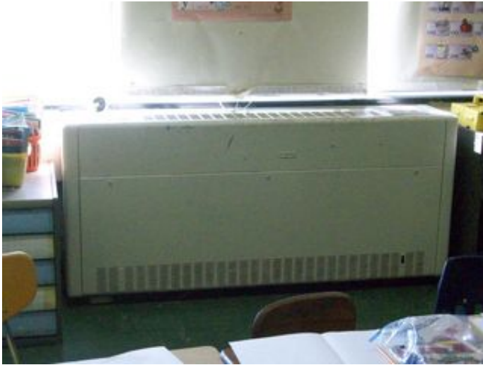
Typical Unit Ventilator
