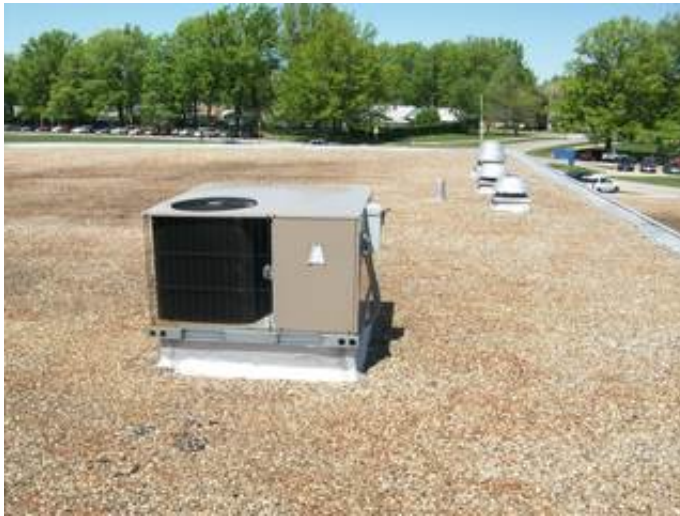
Split Air Condenser Unit & Exhaust Fans
