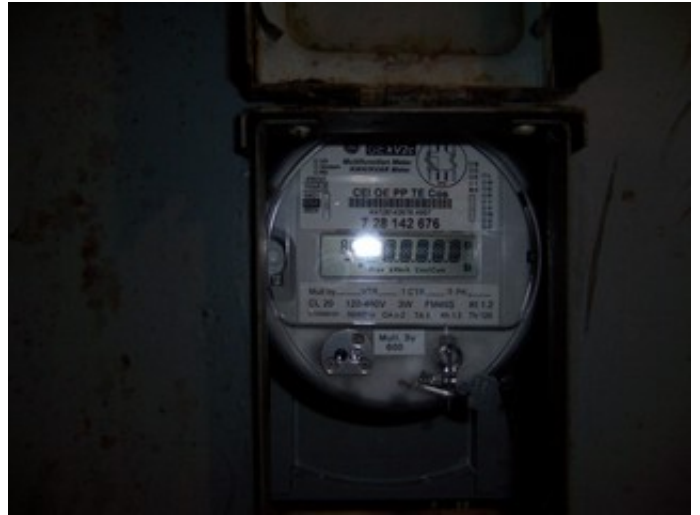
Electric Utility Meter
