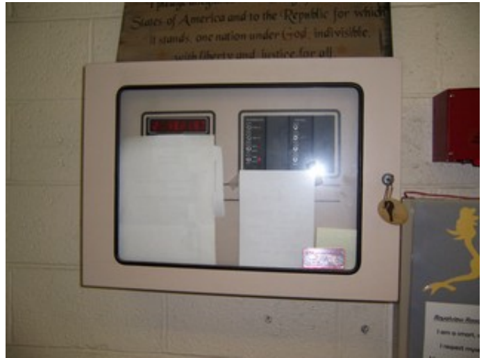
Security System Panel
