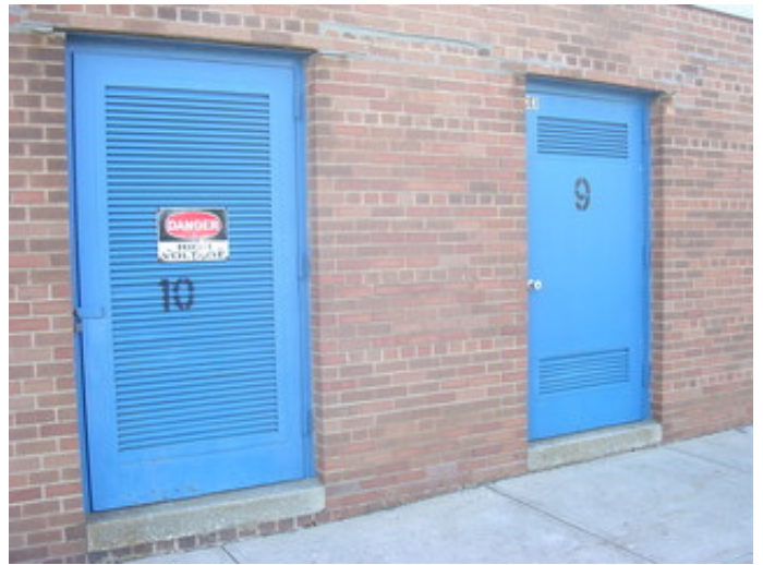
Typical hollow metal doors.
