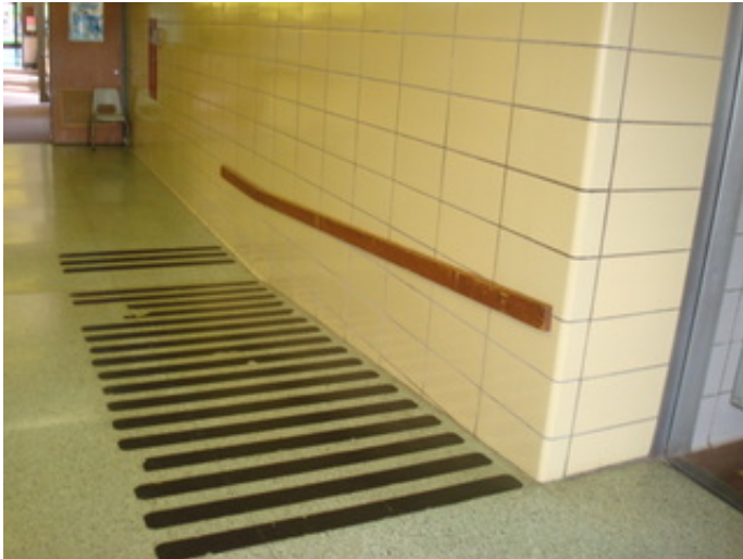
Ramp with non compliant handrail
