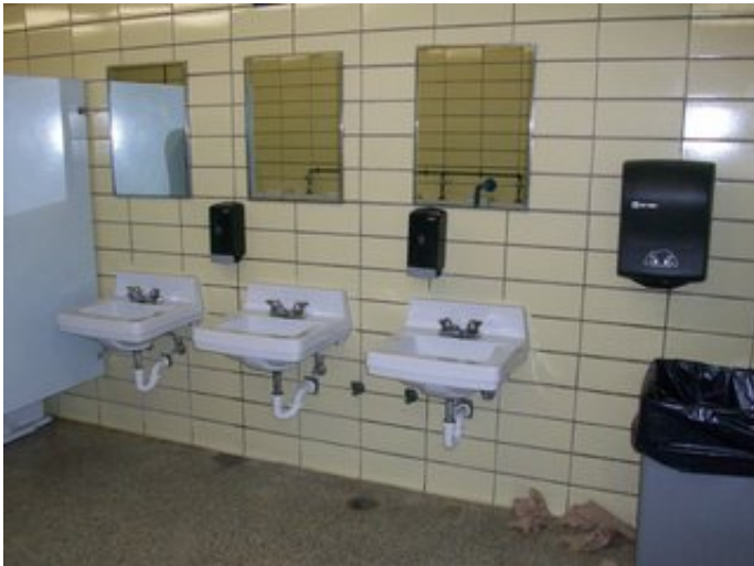
Toilet room fixtures
