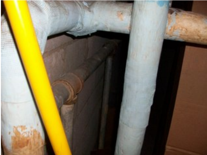
Domestic water in plumbing chase
