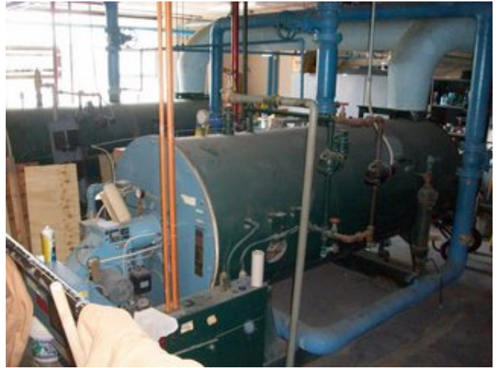
Gas Fired Hot Water Boilers
