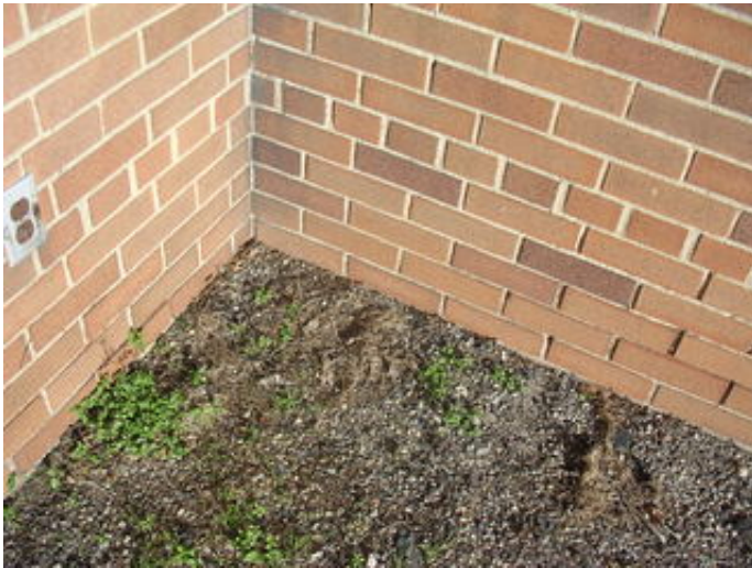
Typical foundation condition.
