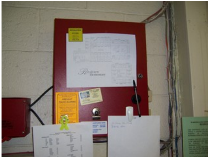
Main Fire Alarm Panel
