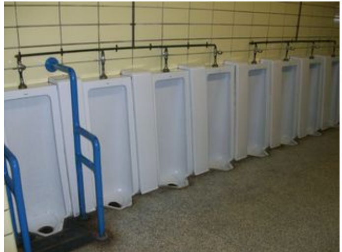
Toilet room fixtures
