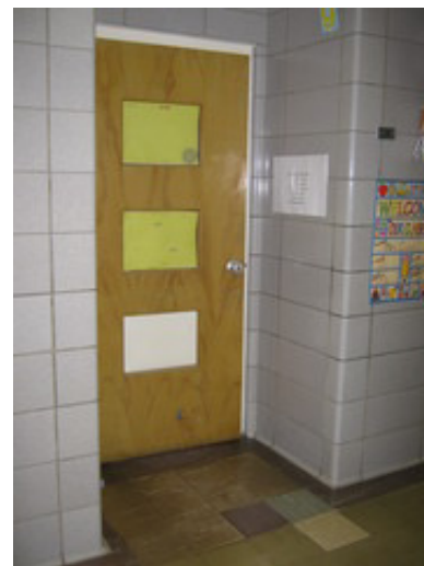
Typical recessed classroom door
