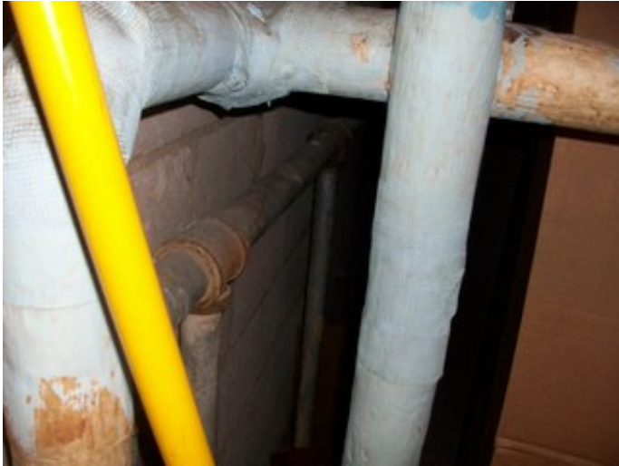
Sanitary drainage Piping
