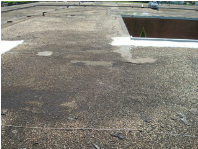
Patched roof over 1956 Original Construction
