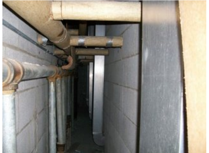
Domestic water in plumbing chase
