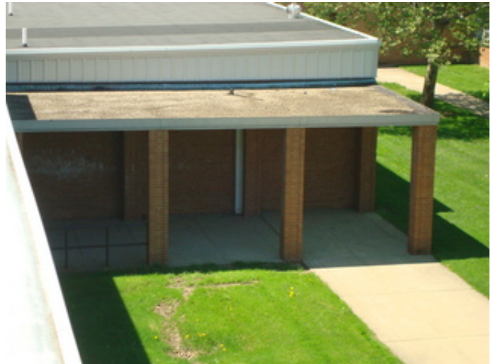
Covered walkway on 1966 Addition
